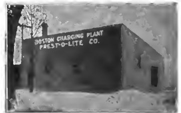
BOSTON CHARGING PLANT
